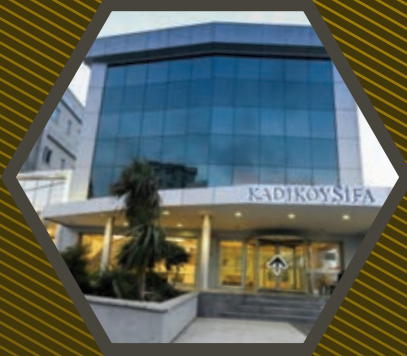
Hopital Şifa Kadiköy, İstanbul Achévé Şifa Hospital Completed
